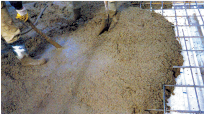
Step 8: Place concrete.
