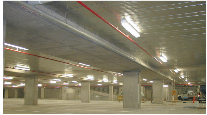
Step 9: Allow slab to cure and remove props.
