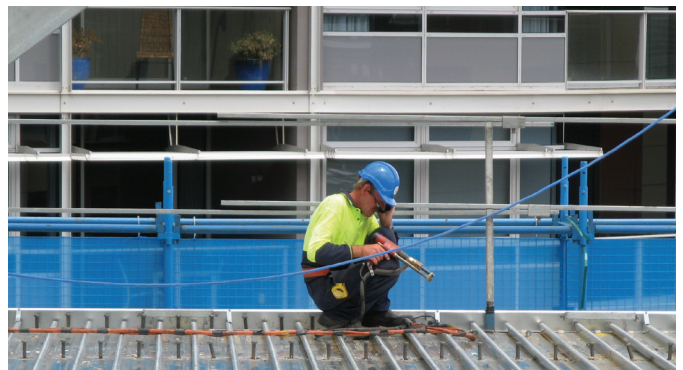
Step 4: Fix BONDEK® sheets to steel beams if required.
