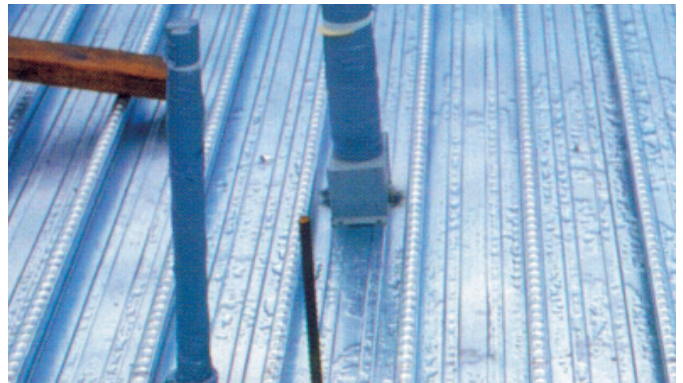
Step 6: Cut penetration.
