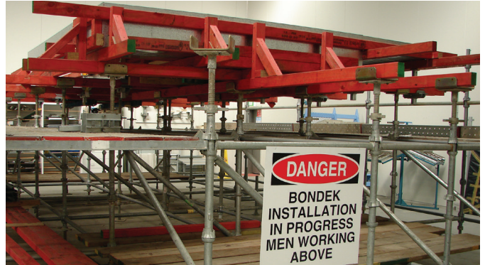
Step 2: Place props if required.
