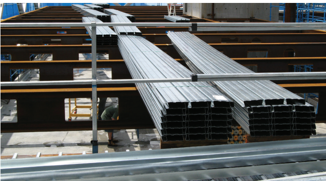
Step 3: Trim BONDEK® sheets if required and place.
